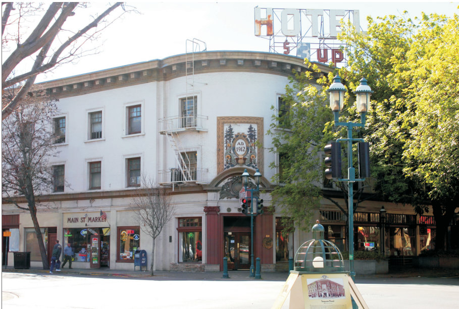
E - 800 Main Street Corner View
