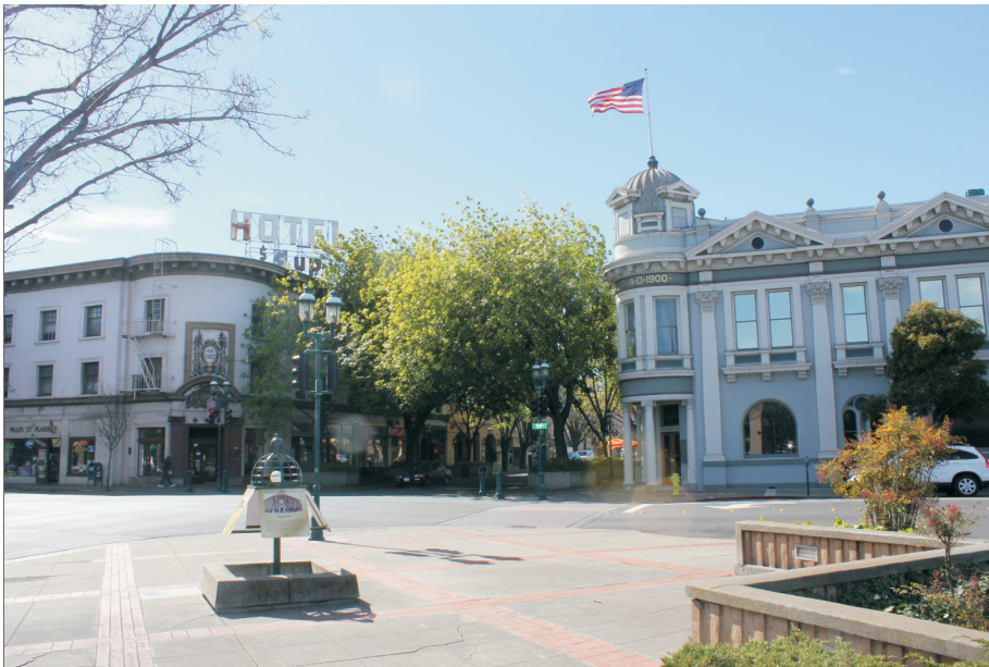
A and E View toward corner of Broadway and Main St.
