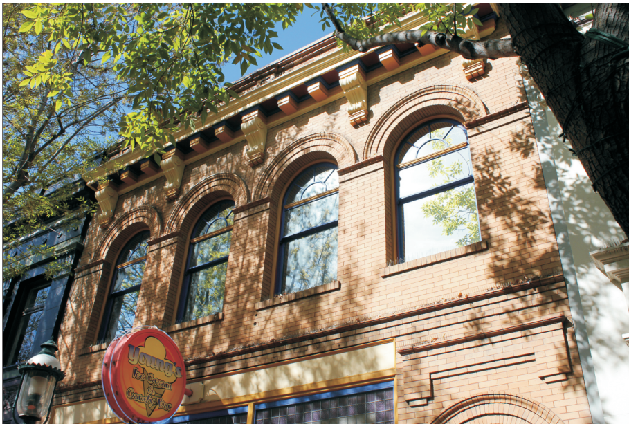
B - 2020 Broadway Window and cornice details
